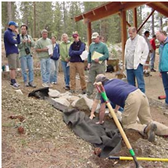
Figure 5. Local contractors learn to install BMPs properly at the annual BMP Workshop. Source: Tahoe Resource Conservation District.
