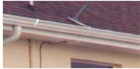
Figure #11: Rodentproofing openings where wires enter buildings.
