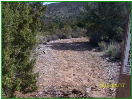
Road before restoration.
