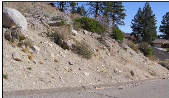
Figure 2. The establishment of vegetation for stabilization on slopes greater than 50 percent is very difficult.
