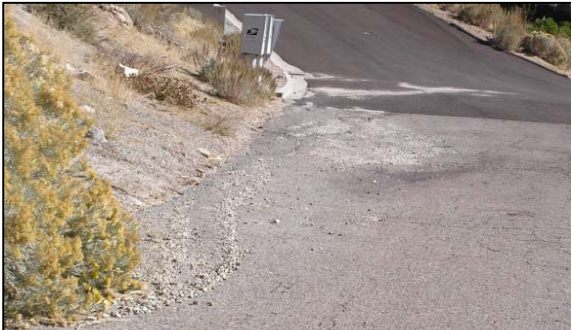
Figure 1. Sediment from eroding slopes can still be seen in the street days after a storm.
