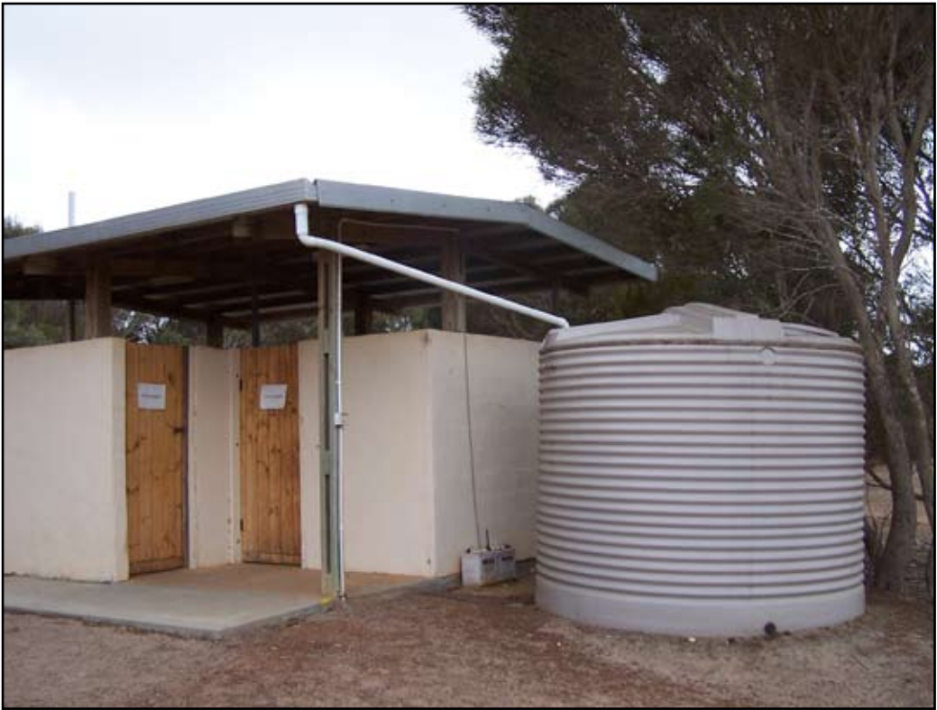
This cistern collects water from the roof of the restroom facility. The water can be used to flush the toilets.
