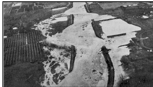
Structures such as levees are not often recommended, as they are known for failing in storms. Walla Walla River, WA. (US Army Corps of Engineers).
