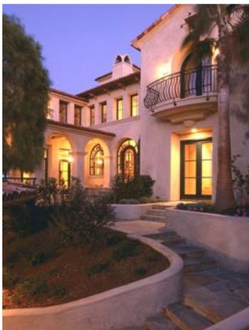
Picture 2. Cement retaining walls surround garden areas. Steps are made of various colored stone. Rod iron railing accents frame balconies and patios. Decorative rock adds color to gardens.
